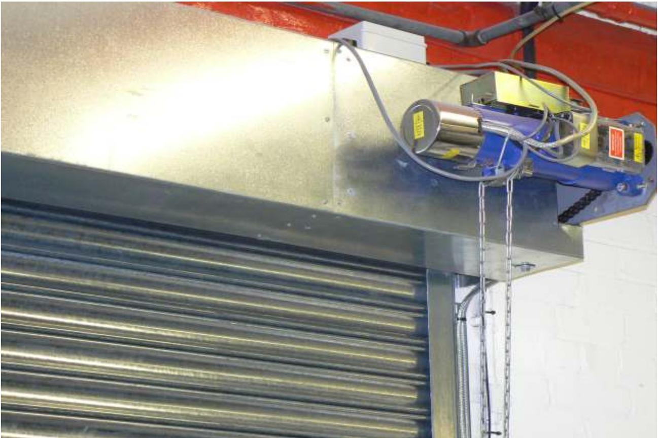
BID Group's Fire Roller Shutters are designed to be robust, providing protection and security whilst providing up to a four-hour delay on the spread of fire in the unlikely event of such a situation. A control descent motor with auto re-set solenoid is fitted as standard.
